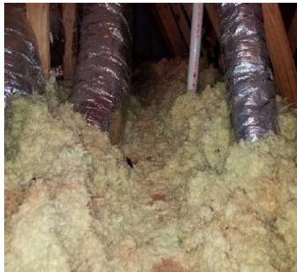
Insufficient Insulation
