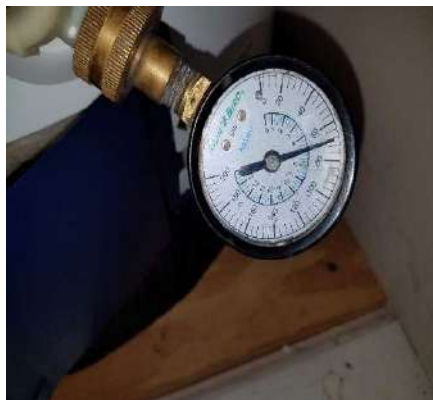
Water Pressure Reading
