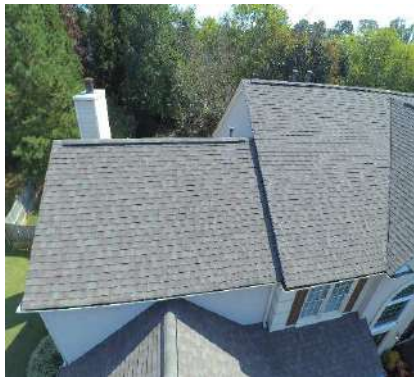
General Roofing Photos
